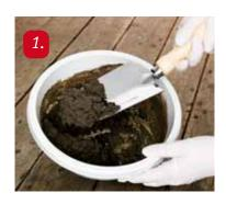
1. Cover your clothes & skin. Mix 1 part water with 5 parts concrete for 5 mins. The mix should look like thick porridge. Add water/concrete as required.
